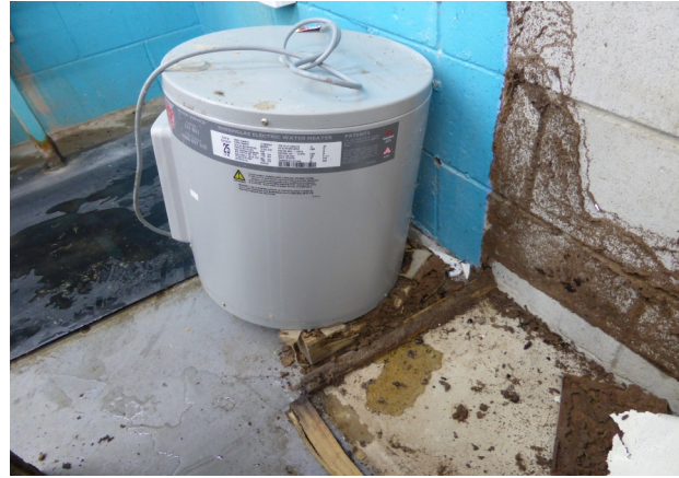
The old Kitchen was riddled with live Termites, The hot water cylinder frame was about to collapse
