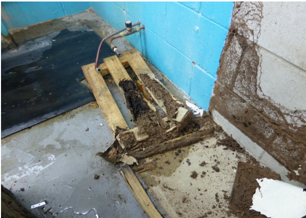
The old Kitchen was riddled with live Termites, The hot water cylinder frame was about to collapse
