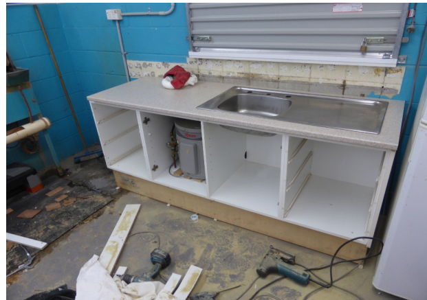
The old Kitchen was riddled with live Termites, The hot water cylinder frame was about to collapse
